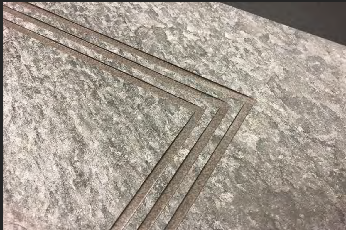
ANTI-SLIP LINES CARRIED AROUND CORNER
